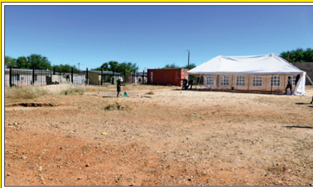
The building site in Katutura
